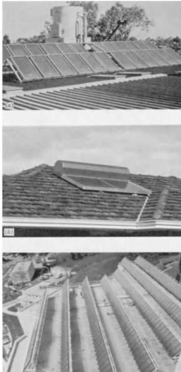
Figure 2.22. Solar water heaters with natural circulation for domestic use and hospitals, and the method of connecting pipes in the cities of Australia. Image source: Affiliated Engineers
