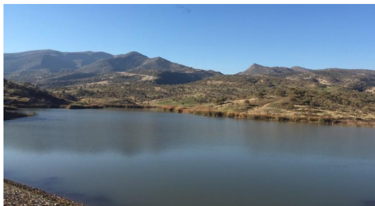
Figure 3.4. General view of the Duhok Dam
