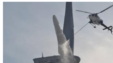
Fig. 2. De-icing task for wind turbine blades. [2].
