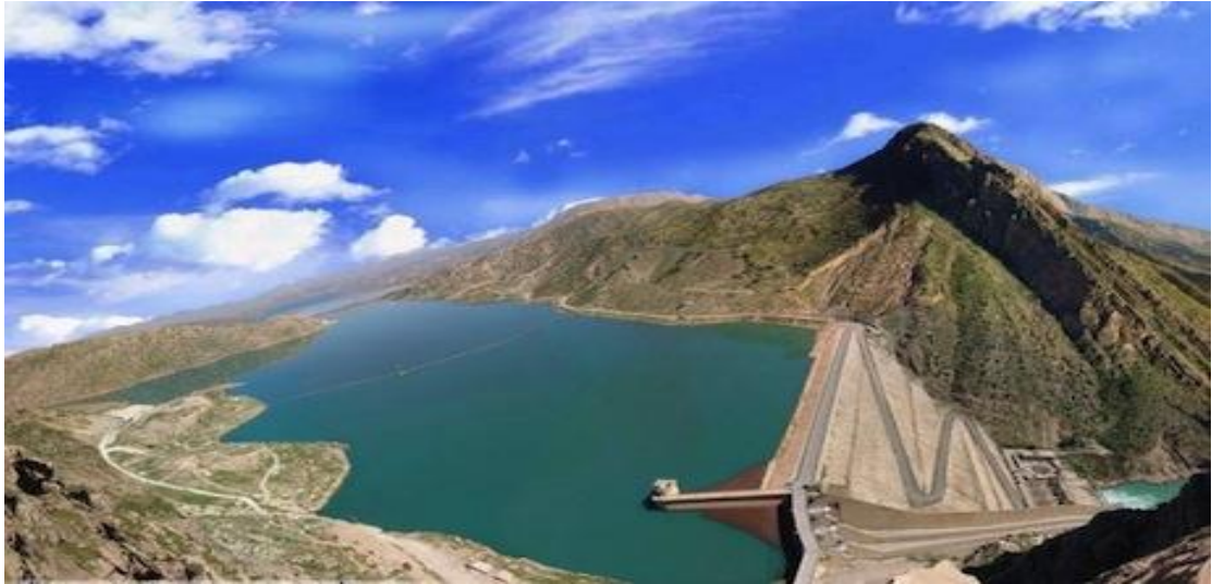
Image 6: Darbanikhan Dam, Sulaymaniyah Province
