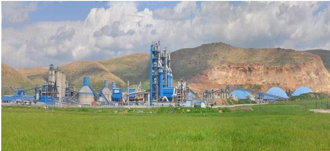
Image 3: MASS Cement Plant- Bazyan
